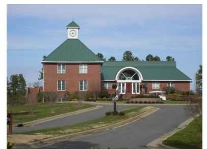
Anderson Creek Golf Club, Harnett County
